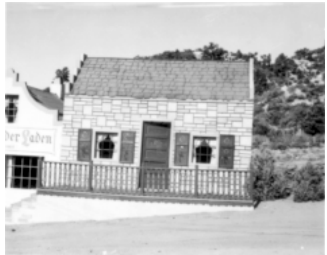
Pat Krig Collection m10009gt.tif Completed Mayor's House. (1944 ca) of a German village.
