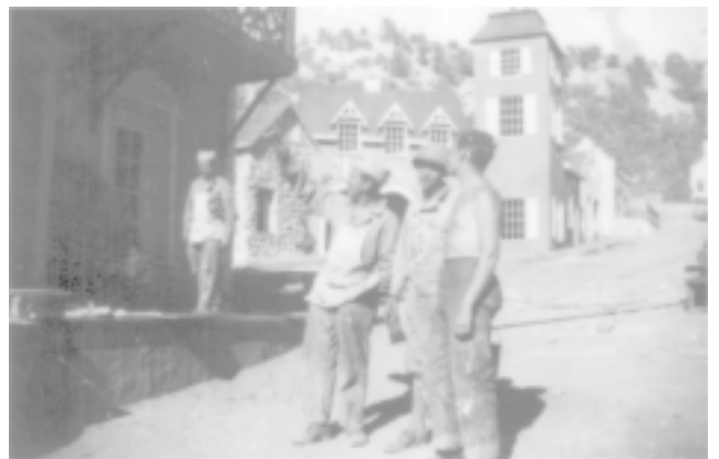
Pat Krig Collection m10037gt.tif Army Engineers Admire Their Work. (1944 ca)
