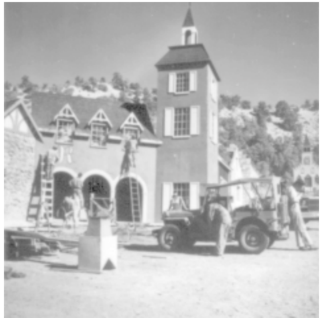
Pat Krig Collection m10018gt.tif Army Engineers Building The Annadorf Town Hall. (1944 ca)
