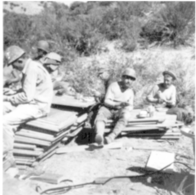
Pat Krig Collection Annadorf Construction Crew. (1944 ca)
