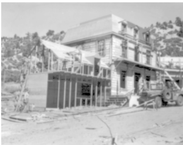
Pat Krig Collection m10030gt.tif "Motel" Construction. (1944 ca)
