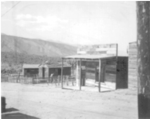
Pat Krig Collection m10027gt.tif Army Engineer Fabricated Annadorf Building. (1944 ca)
