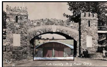
This Garage Roof was used as the form for the Davidson Arch in 1926
