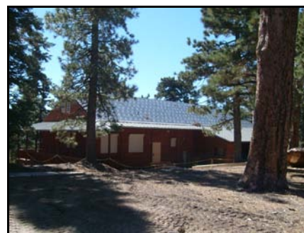
This past year a new metal roof was installed on the Grassy Hollow Visitor's Center
